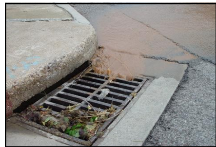
Sediment from a construction site flowing into a storm drain.
